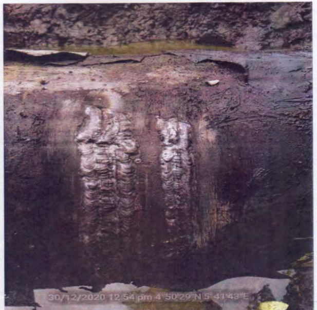
Fig D: Incident facility during repair
